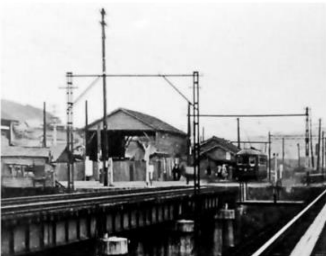
Ohashi-machi Iron Bridge Vicinity
