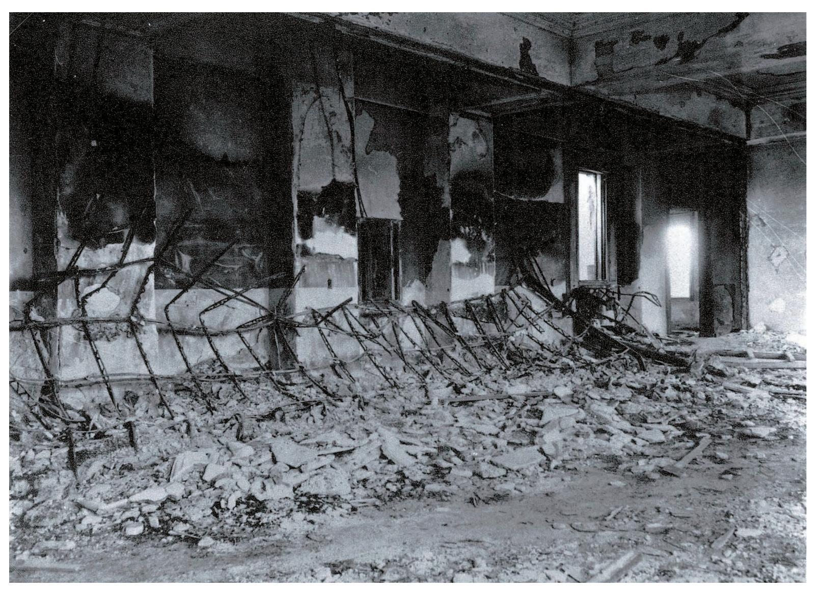
Because the 3rd floor shutter was left open, the whole floor was swept away by the blast wind and the fire.
